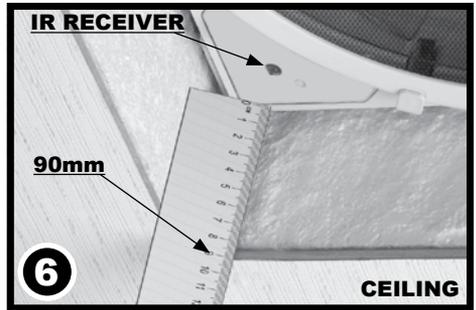
**NOTE:** DO NOT probe or tamper with the thermostat sensor or IR sensor shown in illustration #6 above.
